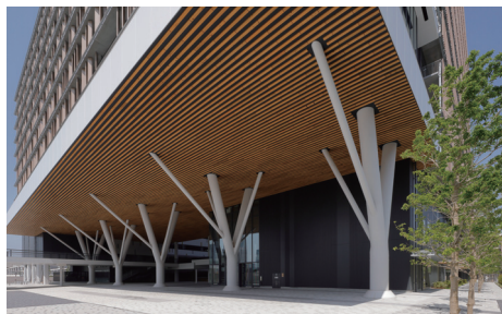
Entrance pilotis featuring tree-shaped columns
