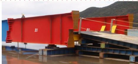
Fig.1 Temporary bridge with end-plate connection
