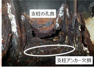
Fig. 2 Damage of steel parapet
