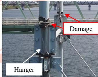
Fig.2 Fracture of suspension material of arch aqueduct
