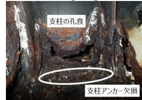
Damage of steel parapet
