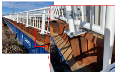
Fig.1 Guardrail post structures for temporary bridges (example)
