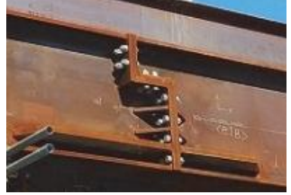
Fig.1 End-plate Connection
