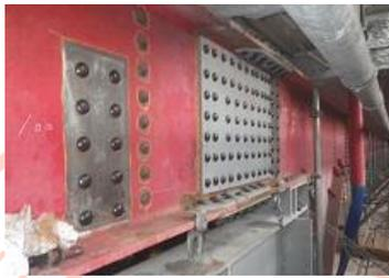
Fig.1 Reinforcement with patch plate
