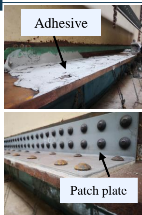
Fig1. Typical patch plate-repair
