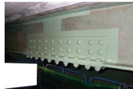
Fig.1 Reinforcement with patch plate
