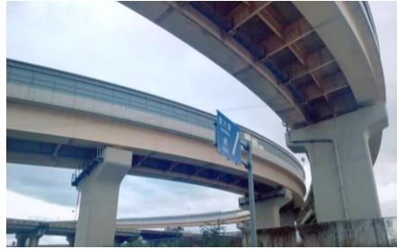
Fig. 1 Steel box girder bridges in urban areas
