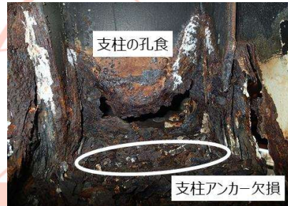
Fig.2 Damage of steel parapet
