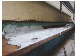
(b) Adhesive for putty lining
