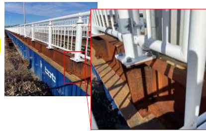
Fig.1 Guardrail post structures for temporary bridges (example)
