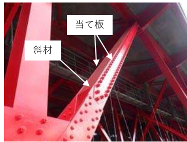
Fig.1 Application of reinforcement using cover plate
