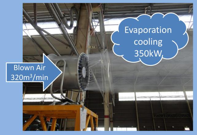
Droplet Sauter Mean Diameter  $d_{32} = 25 \mu m$ Area of cooling with oscillation : Approx. 4000m<sup>2</sup> Daily operating cost (6 fans, water + electric) : 3500yen
