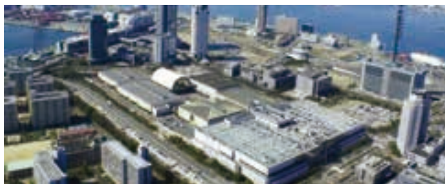
Fig. 3: Trial of the thermal grid at the Osaka International Exhibition Center (1)
